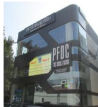
Shopping Complex (2011) Façade New Delhi
