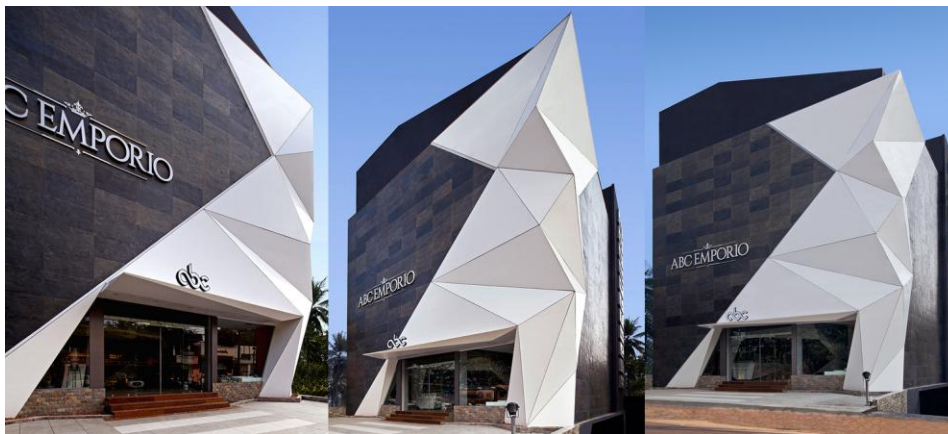
DuPont™ Corian® has been used as exterior cladding partially wrapping the front and the side façade of ABC Emporio in Kerala; Design by NU.DE Architecture; Corian® Fabricator: Genuine Enterprises; Photo by Shamnath J Patil
