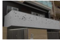
Private Duplex (2015) 3 D cut Balconies New Delhi
